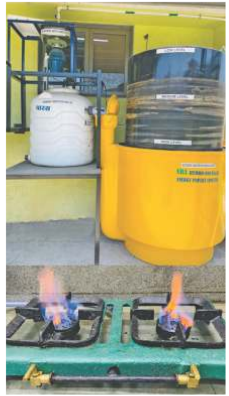
Biogas Plant at Shirwal
