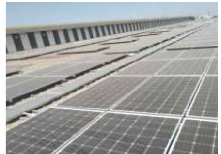
Installation of Solar panel
