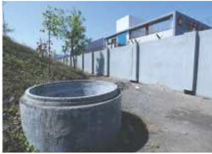
Rainwater Harvesting by Recharge well method
